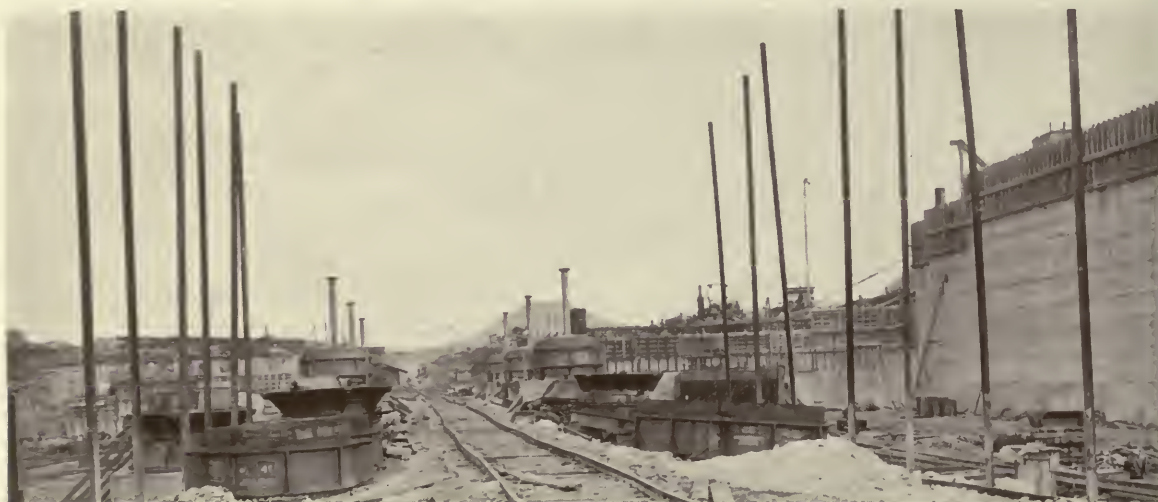
Installing the cylindrical valves for the control of the inflow and outflow of water in the locks.
