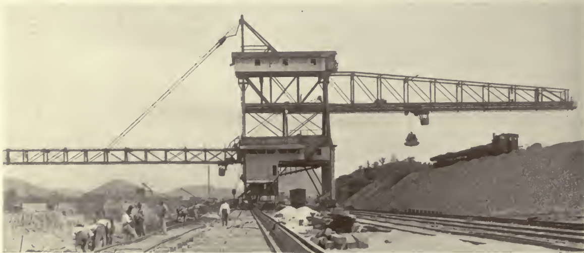
A berm crane in operation. The berm cranes at Pedro Miguel were operated from the head of the lock. The character of the banks at Miraflores made it possible to operate the cranes along the banks. Four berm cranes were used at Miraflores; two set up new and two modified from the ones at Pedro Miguel.
