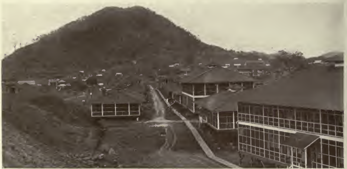
Section East of the Panama Railroad looking North, showing the usual style of buildings. This is in the Pacific Division, where the Pedro Miguel lock overcame a 30-foot difference of level; in other words, connecting the summit or 85-foot level with the 55-foot level.
