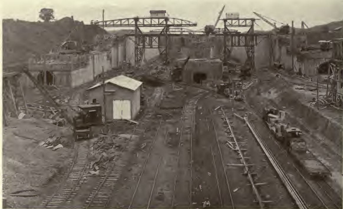
General view of the lock looking South. There are three main culverts extending the full length of the locks, one in each of the side walls and one in the middle wall. These culverts are to fill or empty the locks. The cars convey the heavy buckets of concrete from the mixers to the chamber cranes.
