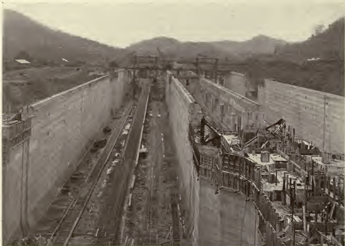
General view of the lock looking North, showing the outer and middle walls almost completed. The steep banks on either side dispense with the arrangement of aerial cableways used at Gatun, hence chamber cranes, shown in distance, are used. Each crane is mounted on four heavy freight-car trucks, which carry it along as the work progresses. All the electrical operating machinery is in the house on top of the tower.
