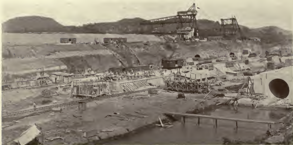
View of locks looking North, showing center and east walls under construction.
